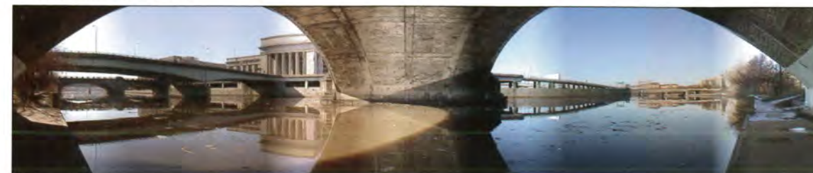
Panoramic from under the 30th Street Station railroad bridge
